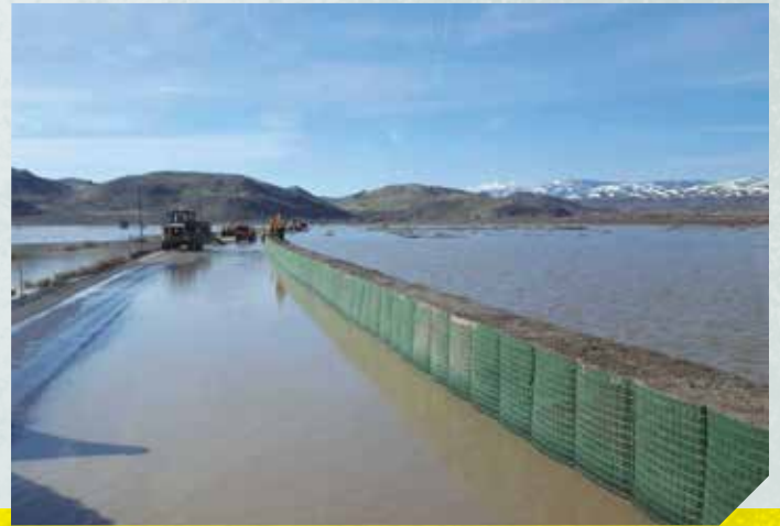
RIGHT: Hesco wall installed by Nevada National Guard members and local first responders.
